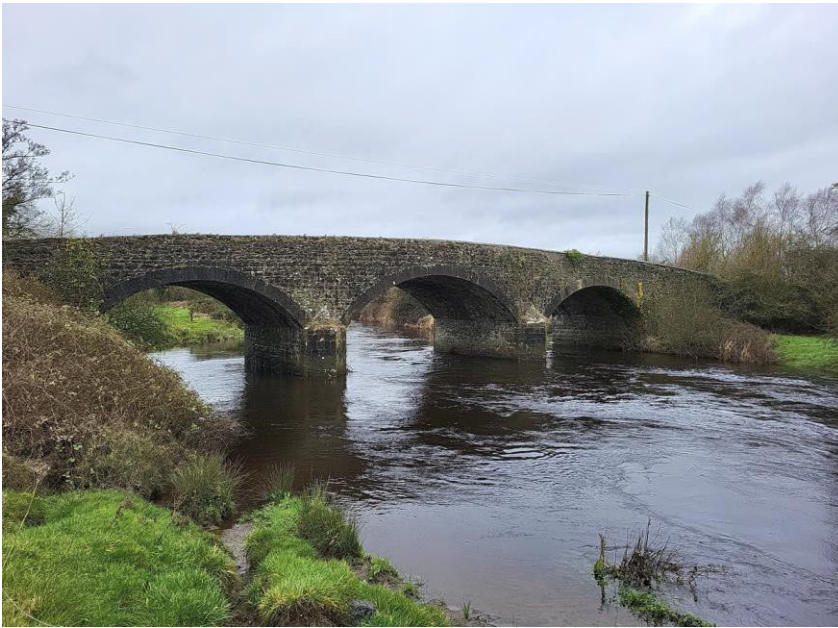
Figure 5.1 – River Barrow Bridge
